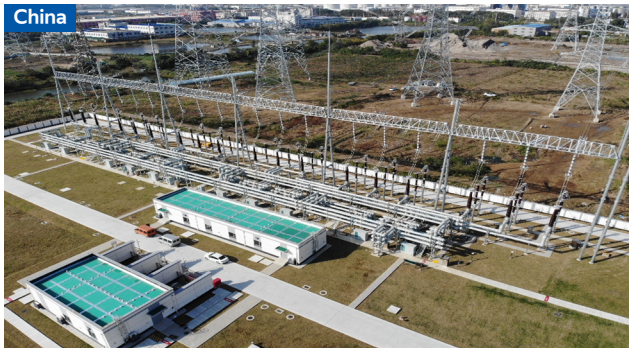
China | State Grid Taohuangang 500 kV Substation Project
