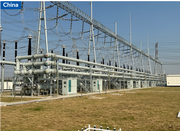
China | State Grid Jiangsu Taohua Port 500 kV switch station new construction project
