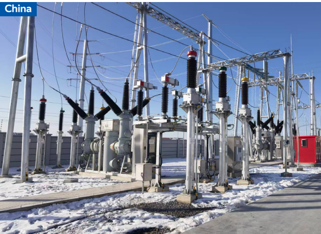
China | State Grid Henan Xinxiang Yuanyangcheng East 110 kV power transmission and transformation project 145kV GIS
