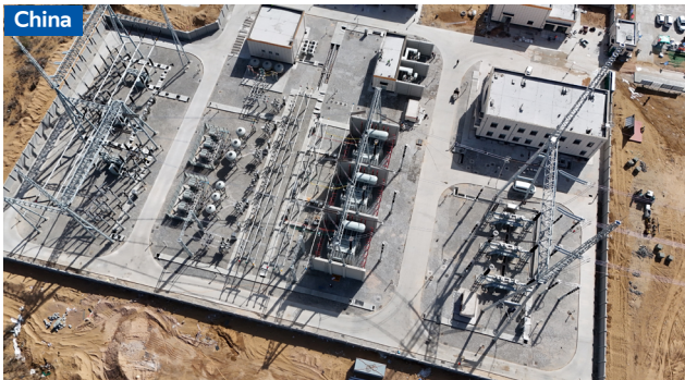
China | Inner Mongolia Power Changcheng 500 kV Substation Project
