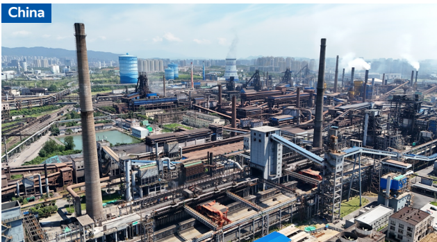
China | Xinyu Iron & Steel 110kV & 220kV Substation Project
