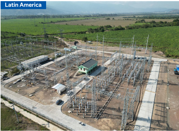
Honduras | ENEE 230kV Substation and Line Expansion EPC Project
