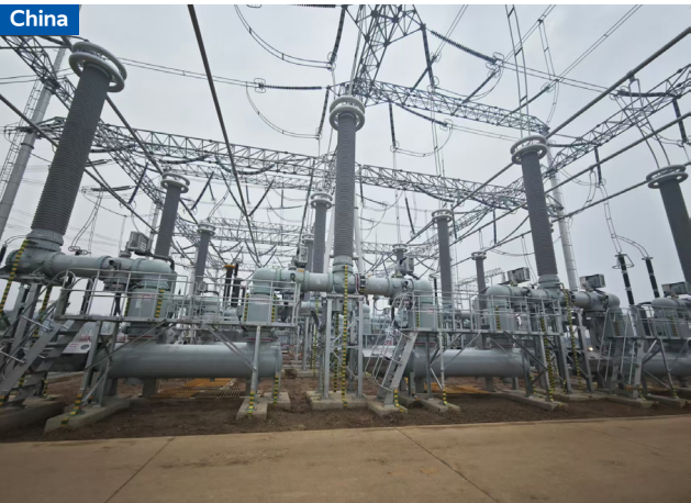
China | State Grid Anhui 500kV Yongqiao Substation 500kV Interval Expansion Project
